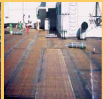
Waterproofing & Joint Sealing
