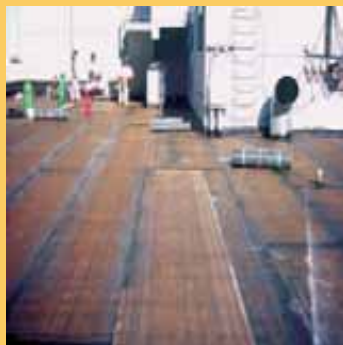
Waterproofing & Joint Sealing
